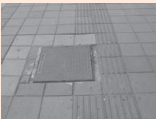
Manhole built on textured pathway on a new street in Belgrade
