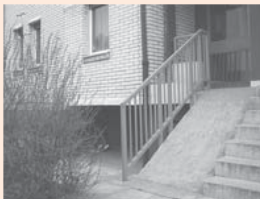
Ramp built in New Belgrade
