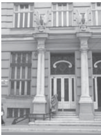
Electronic lift covered due to lack of use in Sarajevo
