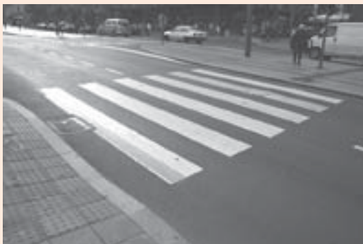
New street in Belgrade, kerbs are not cut on both sides of the street
