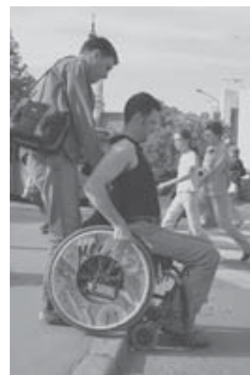
Kerbs are not cut
