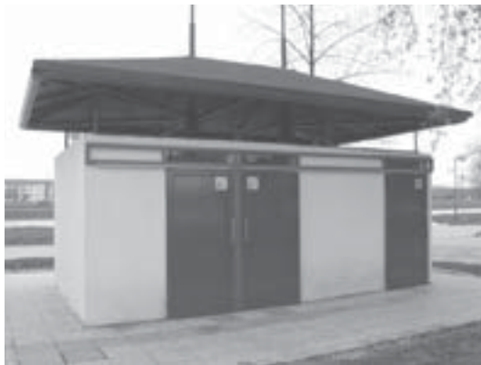
Accessible bathrooms next to regular toilets
