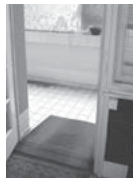
Ramp to the balcony
