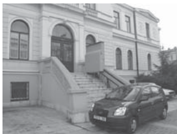
Theatre in Sarajevo, the electronic lift is blocked by a car
